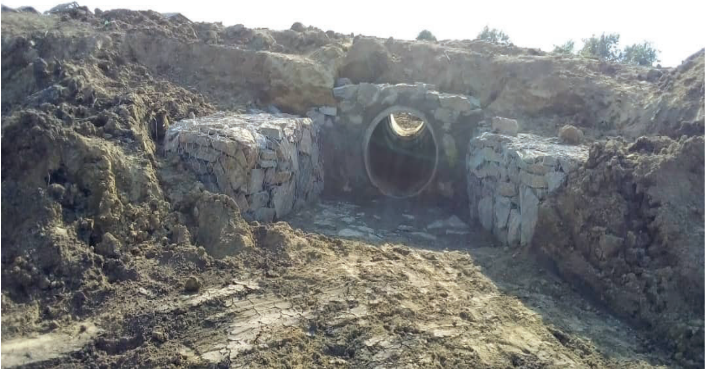
Stone works done for water way
